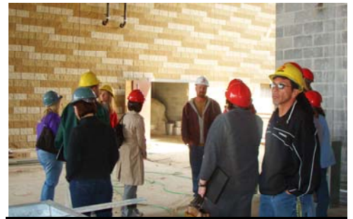
Walking through the construction site for the future Elkhorn High School. Hawkins Construction explained the many diverse trades needed in the construction industry and the opportunities available to students.
